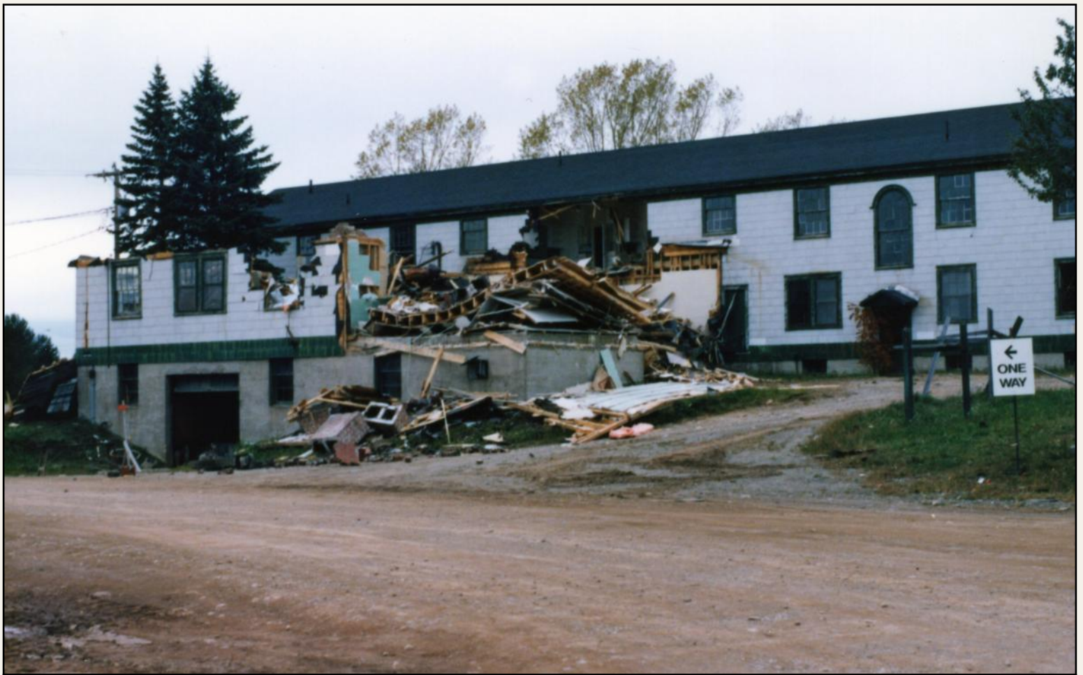
Above and Below: Demolition of Prince Building, in early October 1986.
