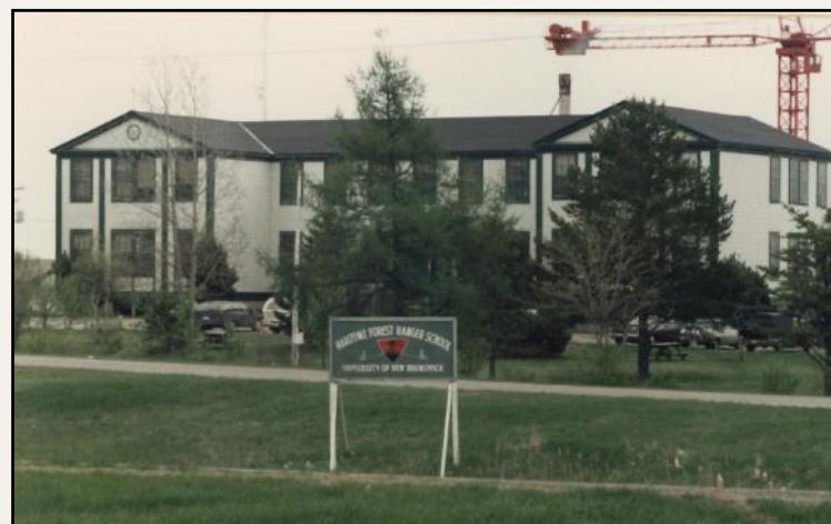
McCormack Building. Administration and academic centre.
