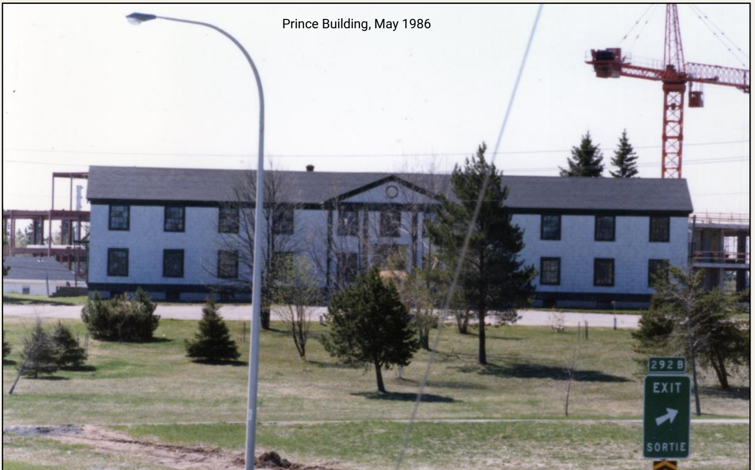
McCormack building, May 1986.
