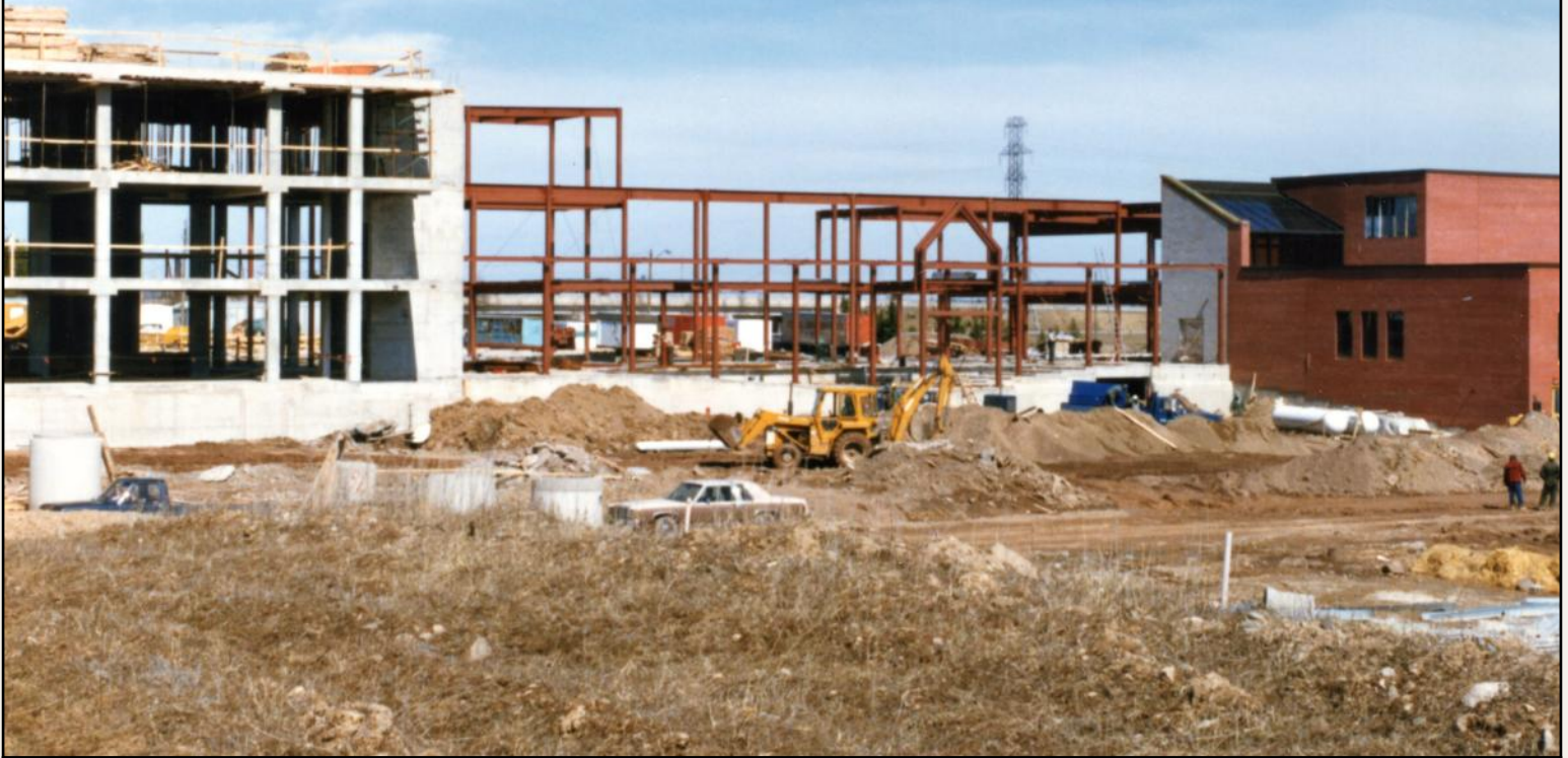
MFRS. Pouring concrete for reinforced concrete pillars. Old MFRS garage in foreground.
