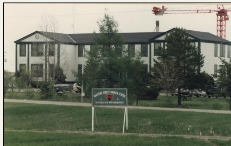
McCormack Building. Administration and academic centre.
