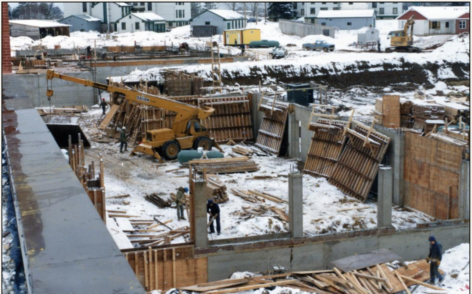
Above: Basement of theatre in the core building January 22nd 1986. Below: Residence #1 looking north, Webb building in background
